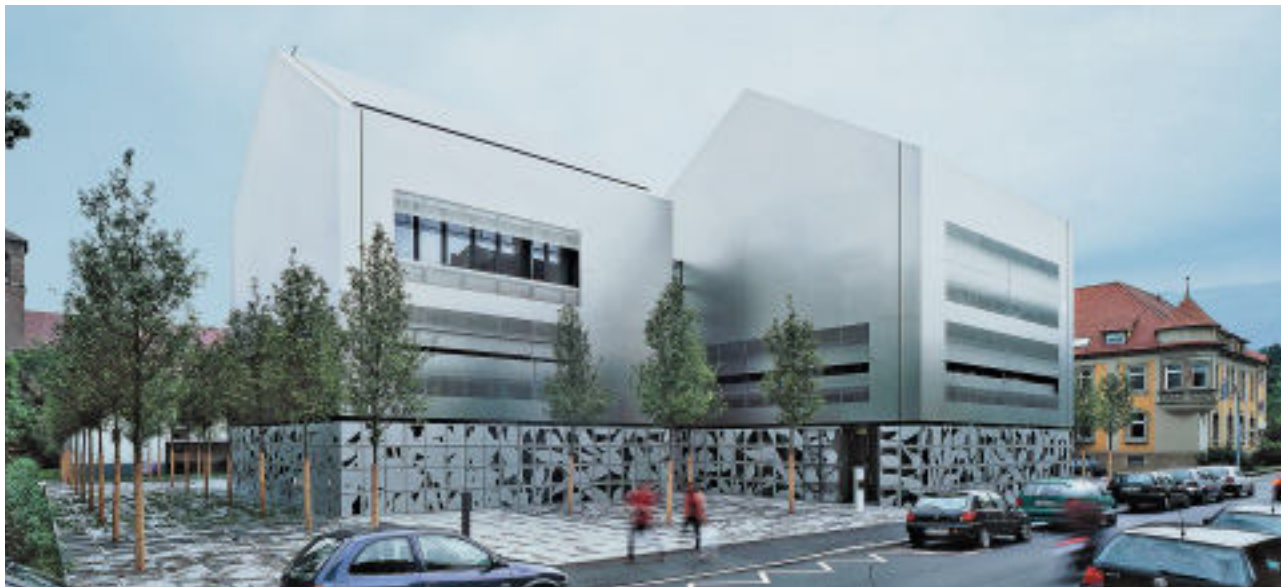
Photo: Florian Holzherr, Munich
