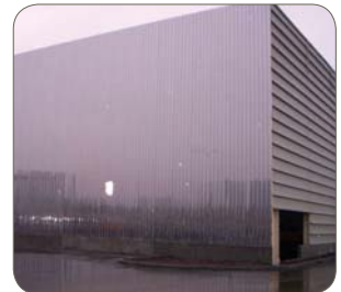
1.4526 (436), Ugine & Alz Steel Service Centre, Arcelor Mittal Stainless, Kattowitz, Polen
